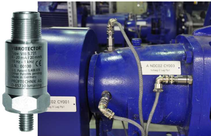
Monitoring vibrations with VIBROTECTOR
